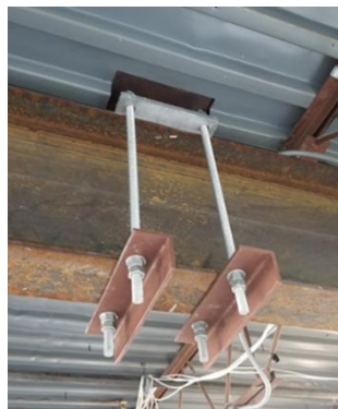
Attached to Structure
