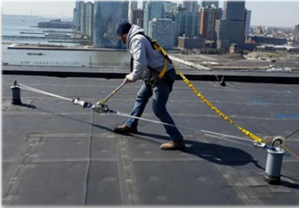
Anchorage Tested Without Measuring Movement
