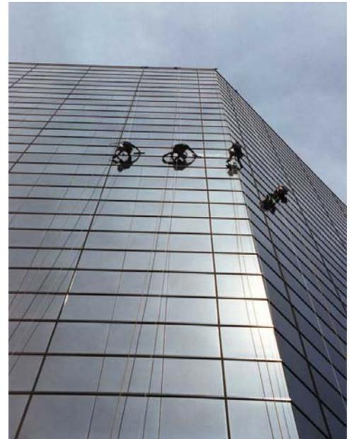
***Bring along an extra RDS to the job. This way if a co-worker does get stranded or needs assistance while suspended, someone can quickly set up this extra system for prompt rescue.***
